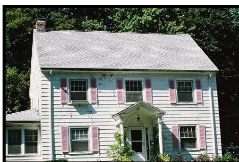
Roof – Next Paint & Windows
