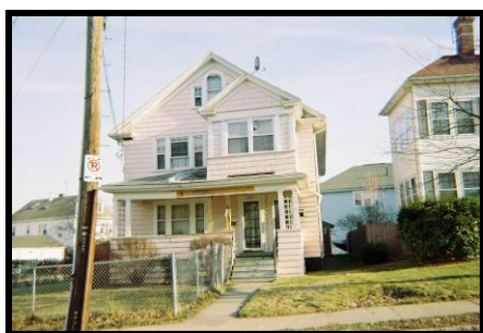
Siding – Windows – Roof & Porch
