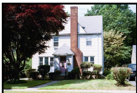
Roof – Gutters – Paint
